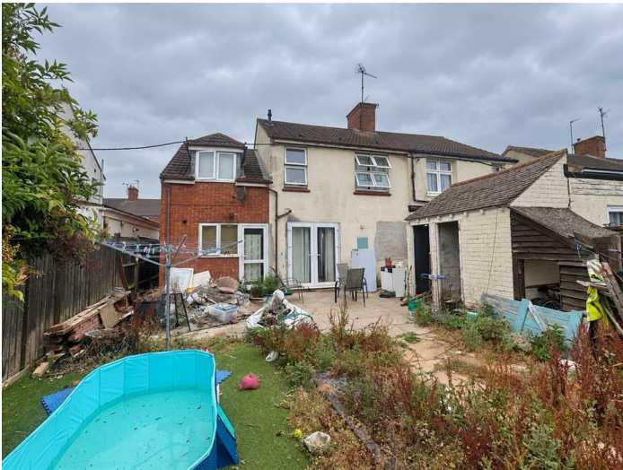
SERVICES / ADDITIONAL INFORMATION Main drainage, water, gas & electrics connected. Users will need to test.
